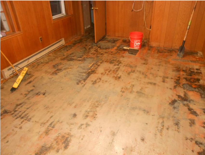
Figure 2: The floor with rug and tiles removed. Here we have most of the black tar removed, but not all. There remains a glue film over the wood, with patches of tar to scrape. The tools used in this job are shown in the picture. The broom helped to push water around and soak it better into the tar paper. A scaper on the end of a large pole was essential.
