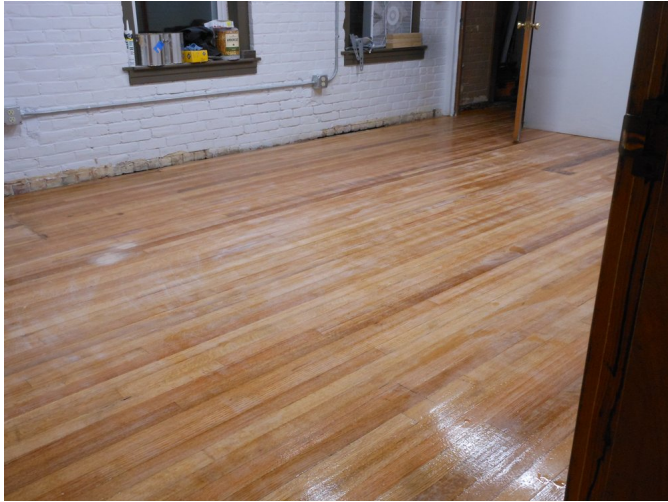
Figure 12: The floor with two coats of urethane, and then sanded with a handheld orbital. The white blemishes, are from sanding. A floor orbital would've been easier, but even with a handheld, it's no more than two hours of work (60 grit).
