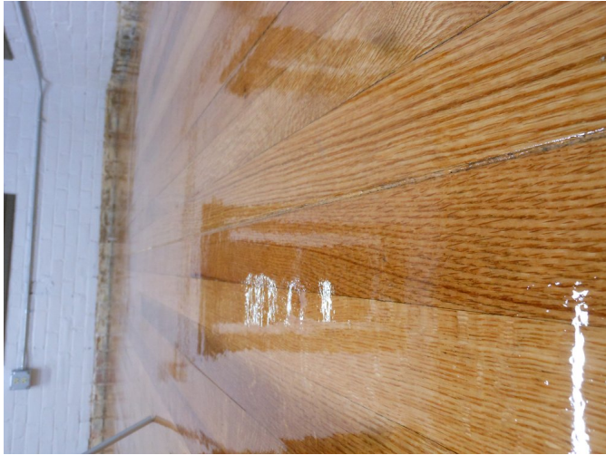
Figure 15: The Aliphatic Urethane is a glossy urethane. Three coats were required to get a smooth finish.
