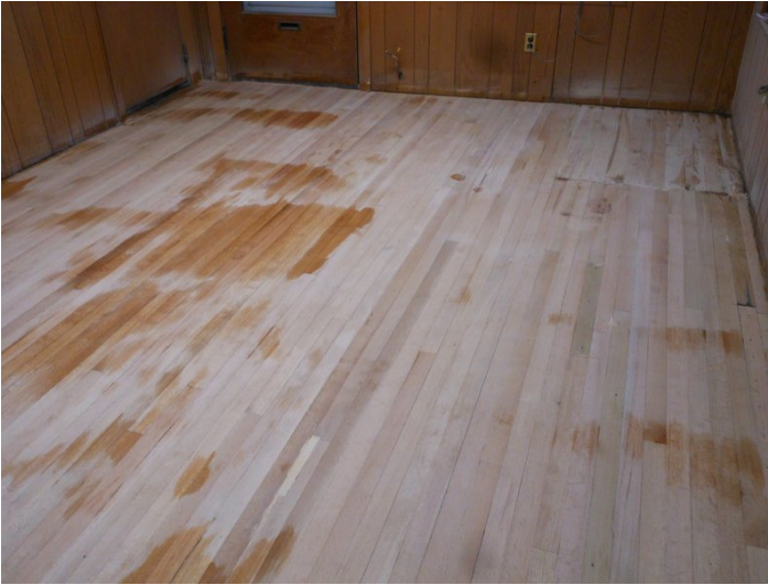
Figure 9: The floor should be cleaned well before applying finish. Any dust left on the floor will remain under the finish as well.
