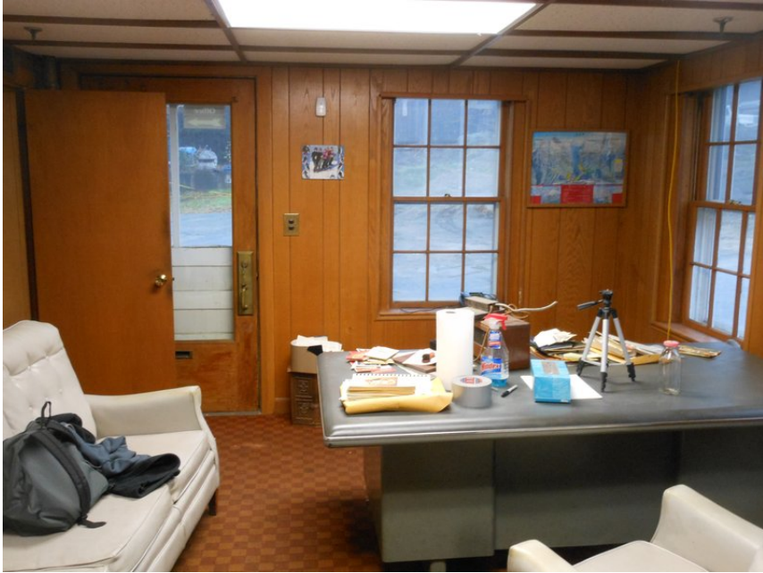
Figure 1: Room Before Renovation: The rugs are difficult to clean. The drop ceiling hides the all wood joists / subfloor above, and the walls are dark / dusty. This project started, as a desire to remove the rugs, but led into renovating the remaining aspects of the room.
