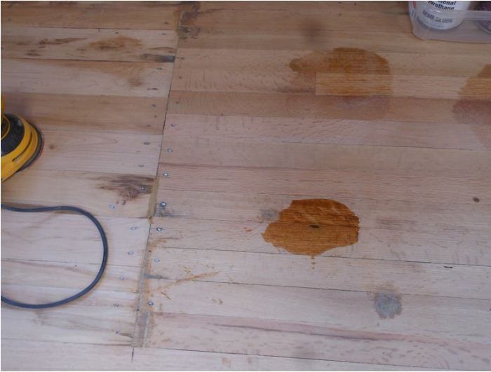
Figure 8: Here you can see wood glue appear dark, under the finish.
