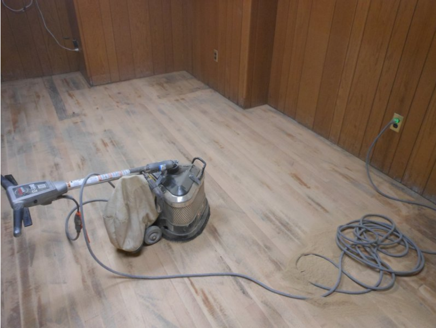
Figure 3: The orbital sander did not fully sand the floor.
